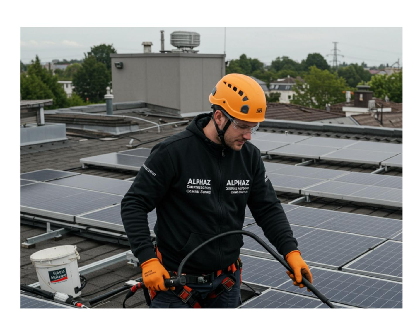
Solar panels must be clean and damage-free to operate efficiently. Bird droppings, dust, leaves, and pollution can block sunlight and reduce power output by up to 25%.
